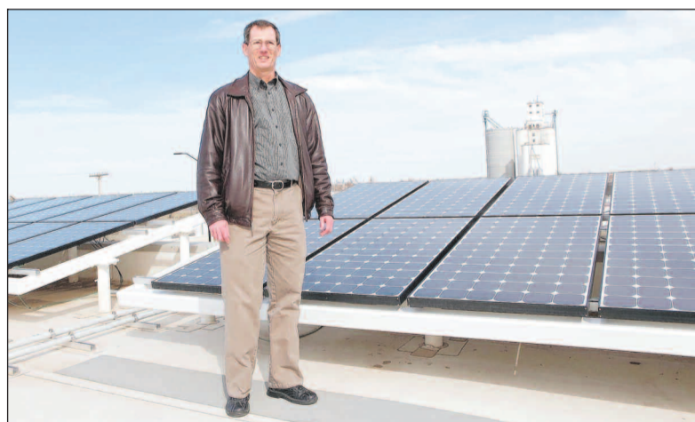
Jaime Green/The Wichita Eagle Solar panels on top of the Business Incubator building are one source of energy. Tim Lenz of Professional Engineering Consultants helped design the building and many others in Greensburg.
